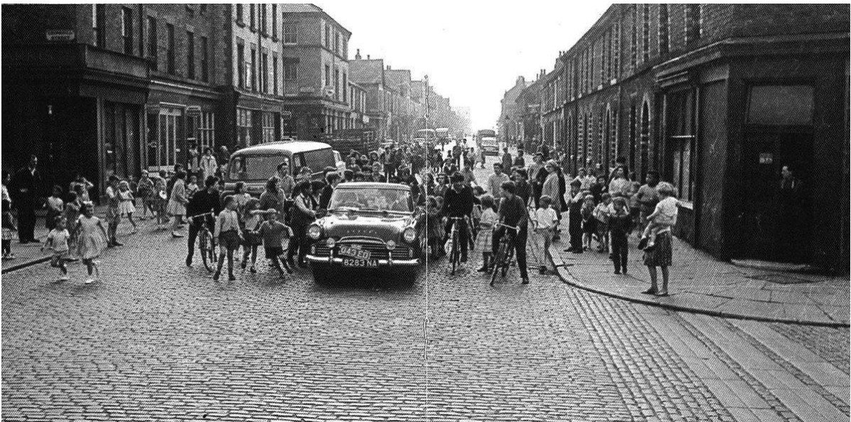
This photograph, showing Ringo arriving back in Toxteth in the 1960s [included as an insert in his 2008 album 'Liverpool 8'], demonstrates the subsequent erosion of the character of the area, not just in terms of the street frontages and density, but also the surfaces of the streets and pavements [which are now mostly tarmac].
